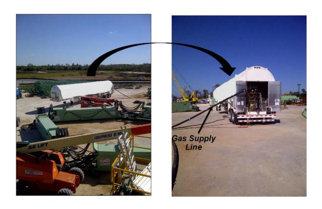
Figure 3 LNG Storage Trailer
