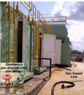
Figure 4 Generator House, Gas Supply Lines, and Shut-Off Valve
